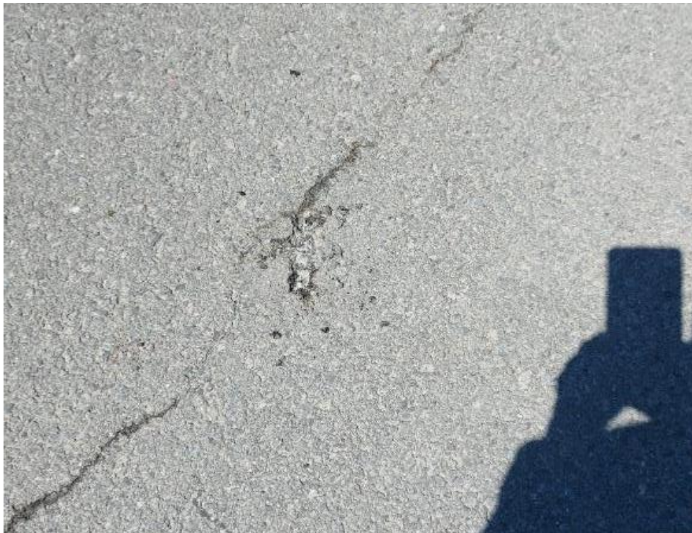
Photograph 16: Bridge No. 16-166 – Highway 401 Merwin Lane Underpass. View of bulk asphalt sample 16-166-ASP-01A along top side of the bridge. All bulk samples collected from the Site found not to contain asbestos.
