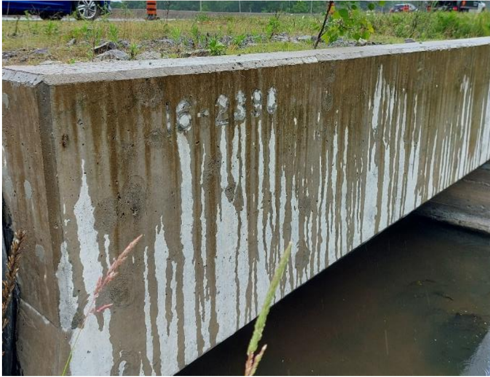
Photograph 53: Structural Culvert 16-239/C – Highway 401 Lemmon’s Creek Culvert. View of culvert stamp with construction date along the east side of the culvert. Culvert stamped 16-239C.
