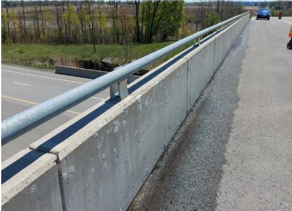
Photograph 15: Bridge No. 16-166 – Highway 401 Merwin Lane Underpass. View of concrete barrier wall with single metal tube railing along the west side of the bridge.
