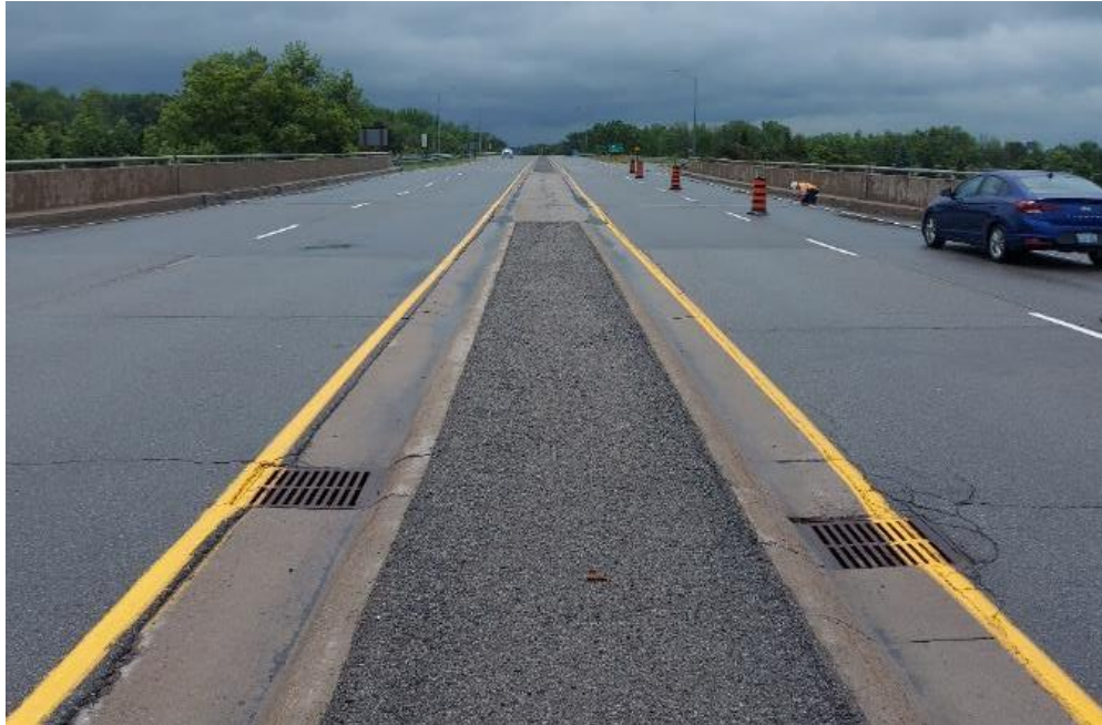
Photograph 43: Bridge No. 16-130-Highway 16 U/P. General view looking south along the bridge.
